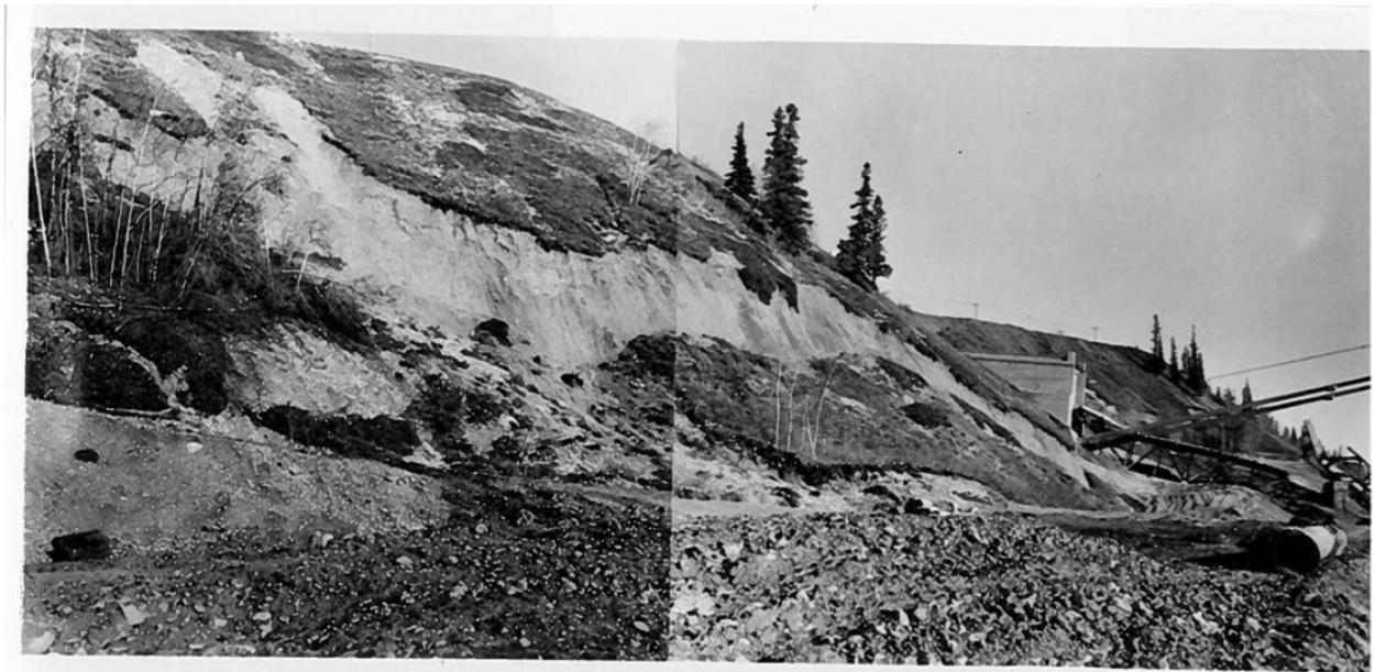
Figure 3. View from west of scarp of landslide, North abutment and collapsed approach span in background
